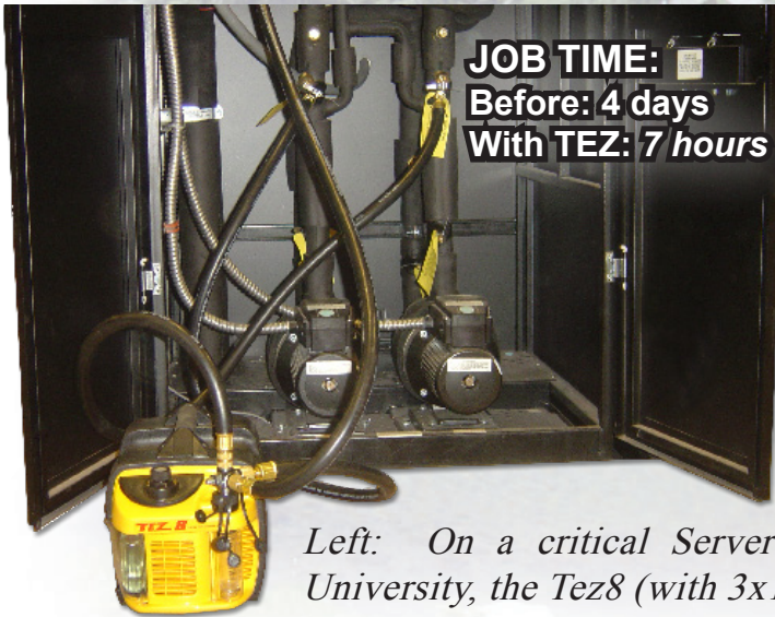
Above: With five simultaneous connections, the TEZ Speed System evacuates racks like these up to 10 times faster than typical vacuum pumps.
